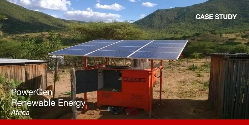
PowerGen Renewable Energy implements hybrid power systems with solar, battery storage and generator back-up to supply electricity to underserved communities where grid expansion is not an option. PowerGen has established microgrids in over 120 communities across Africa, with New Sun Road's technology providing remote power management solutions to ensure seamless operations and optimization of its power assets across the continent.
